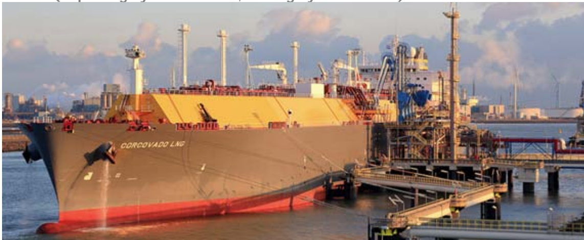
The 294 mtr long 2014 built CORCOVADO LNG moored at the Rotterdam GATE terminal
