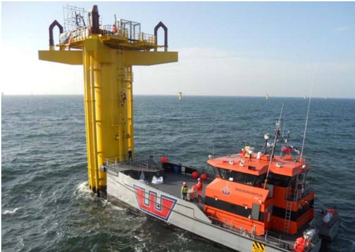
The OFFSHORE WIELINGEN operating at the operations at the Luchterduinen Windfarm in the Netherlands.
