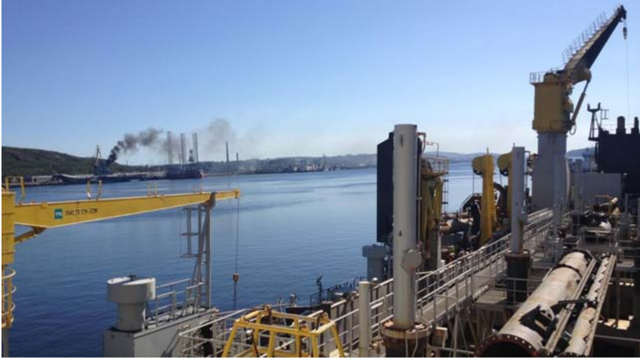
Jan de Nul's AL IDRISI operated at the Port Sabetta project - Photo : Bart Brusse ©
