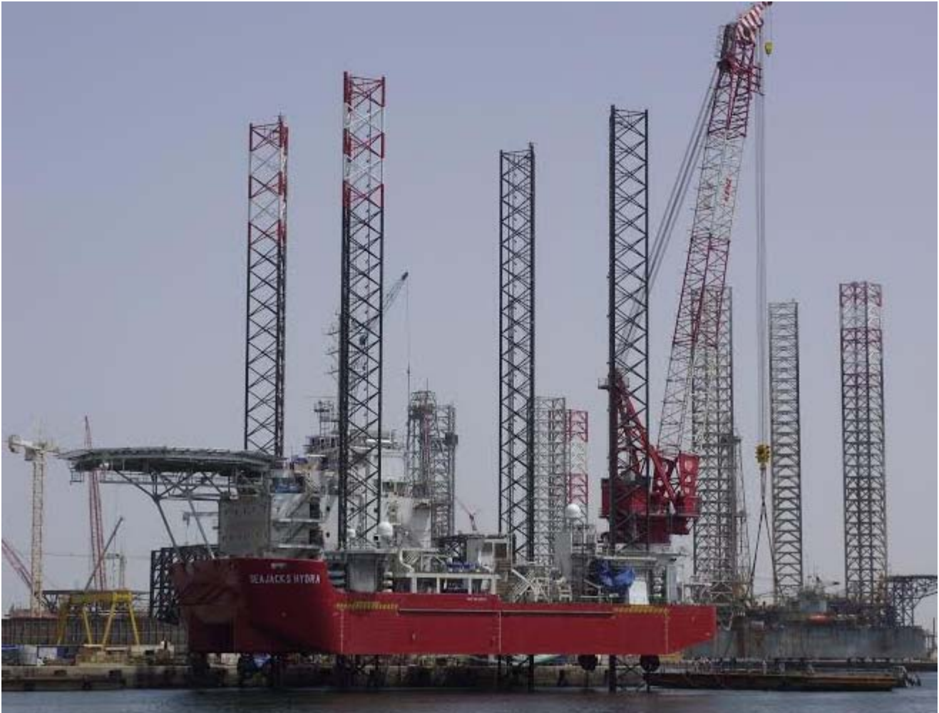
25-03-2014: SEAJACKS new build HYDRA seen during the overload tests off the Dutch made 400tons Kenz-crane At Lamprel's construction yard in Sharjah, United Arab Emirates.
