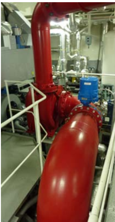
Two seawater centrifugal pumps, each capacity of 1760m 3 /hr @ pump speed of 1800 RPM are installed in the engine room and are driven by the main engines
