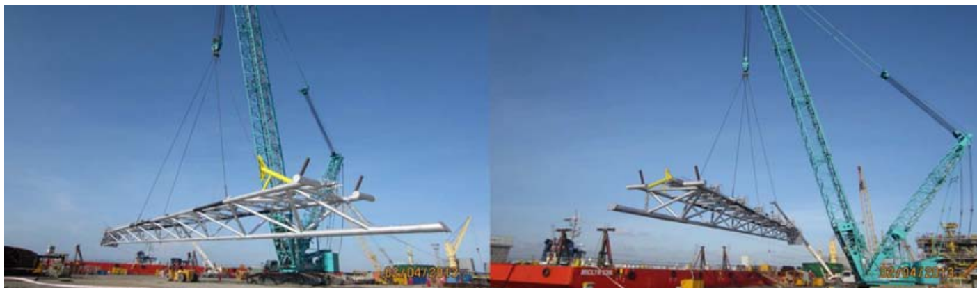
02-04-2013 : The HST (Hai Su Trang) field flareboom loaded out at PTSC yard in Vungtau Photo Capt. Jelle de Vries
