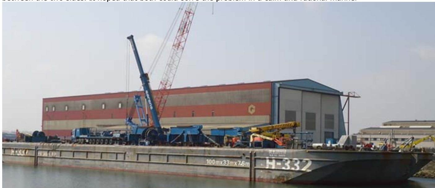
Sarens positioned a small dozen of winches and is assembling the first level of the support structure on one "H-332" of the two barges for the installation of the new bridge "De Oversteek" in Nijmegen. Photo : Ben Duym ©
