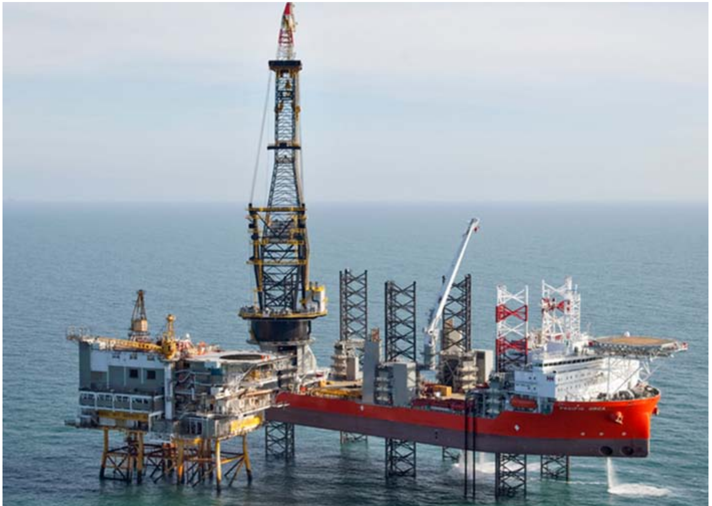
The PACIFIC ORCA installing the H7 platform at the Bard Field photo : FLYING FOCUS luchtfotografie - www.flyingfocus.nl (c)
