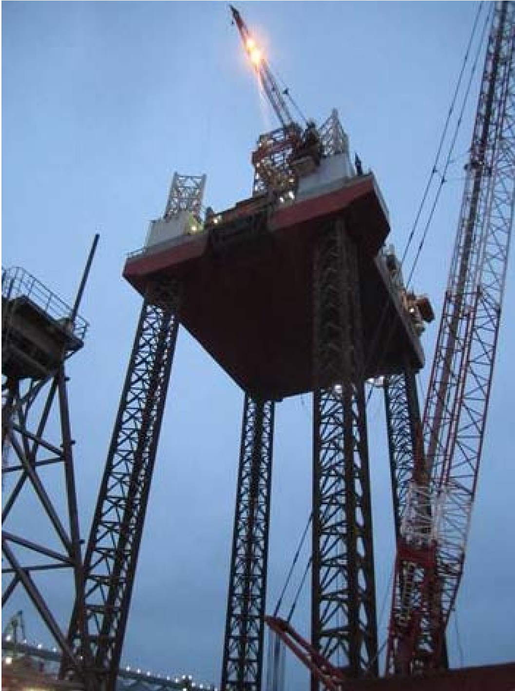
Seen in Constanta, Romania at the GSP (Grup Servicii Petroliere) yard . Maintenance and shortening of legs Jack-up rig GSP JUPITER photo : Henk Willemsen ©
