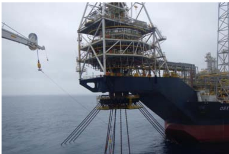
The transfer of raisers layed by AKER WAYFARER on the seabed to the FPSO OSX 3 at the Tubarao Martelo Oil Field in Brazil. Photos : Sondre Butler Gangdal ©
