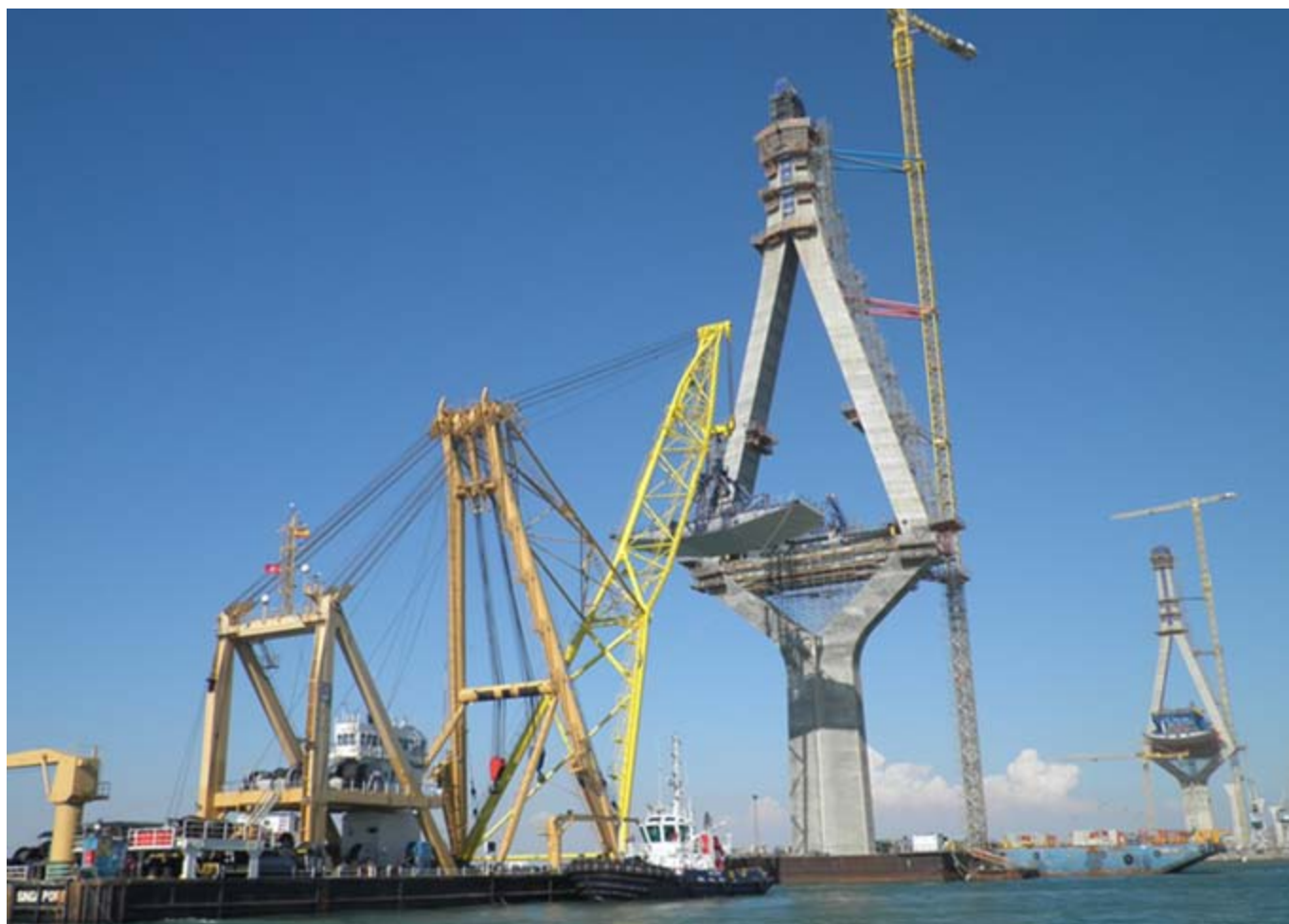
The sheerlegs TAKLIFT 6 equipped with 100m longboom, installing a part ( 385 mT, 60 m over the sea level) of the to be built Puente sobre Bahía de Cádiz. Photo : Antonio Fernandez Acosta ©
