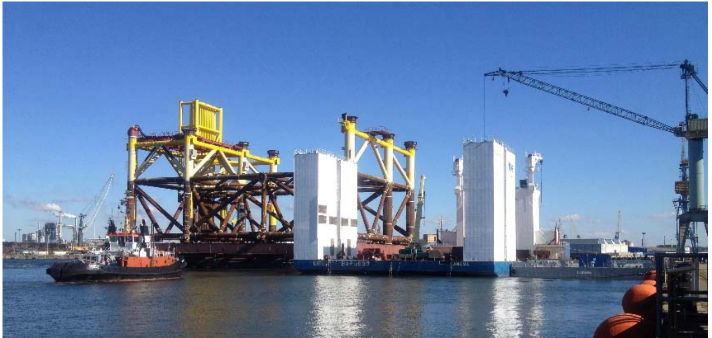
Skidding 7750 mTon from the H331 barge to the submersible barge Eide 33 by Mammoet in Wismar, Germany
