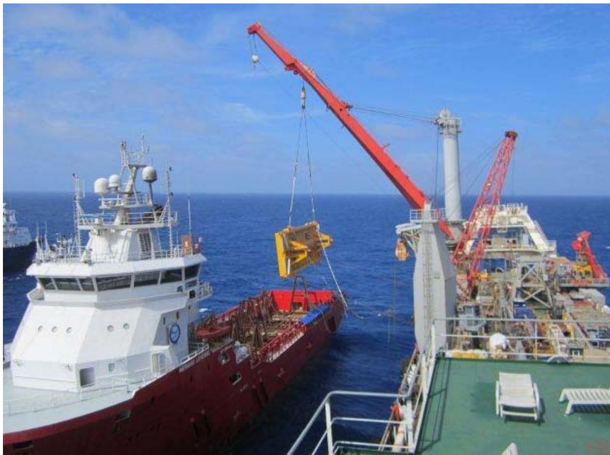
The last APS-lift with weight of 120Mt by LORELAY from the MERMAID LEVEQUE At the Gorgon Jansz field located NE of Barrow island NW-Australia, the APS will be installed at the seabed at a depth of 1300 mtr Photo : Capt Ruud Matthes -Master "Lorelay" ©
