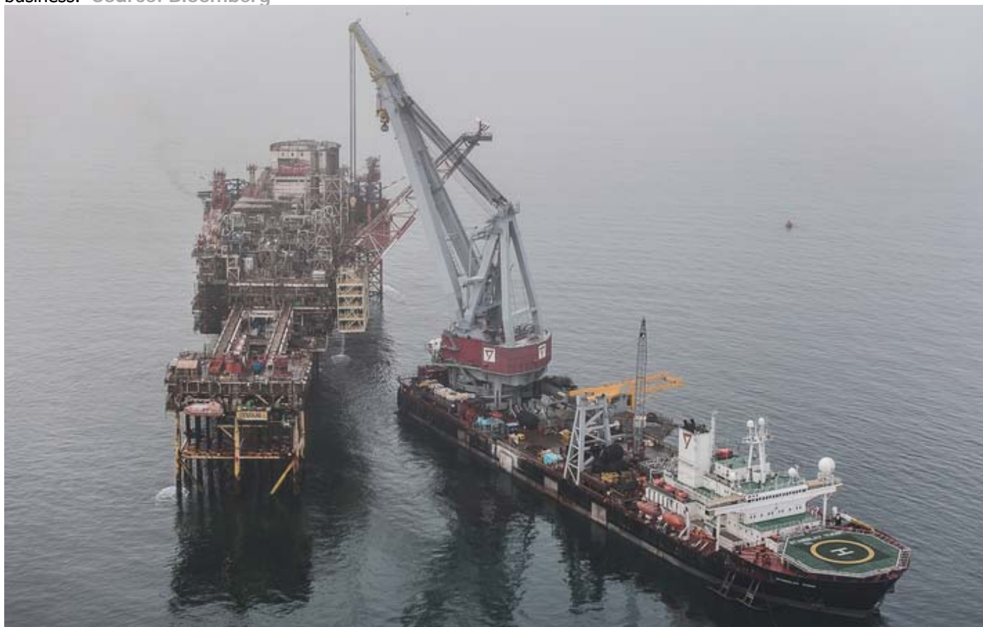
The STANISLAV YUDIN operating at the Douglas Platform in the Irish Sea where the Seaway heavy Lifting crane vessel installed a 270 ton in weight module (20 x 7 x 14 meter) on the outside of the existing Douglas Platform
