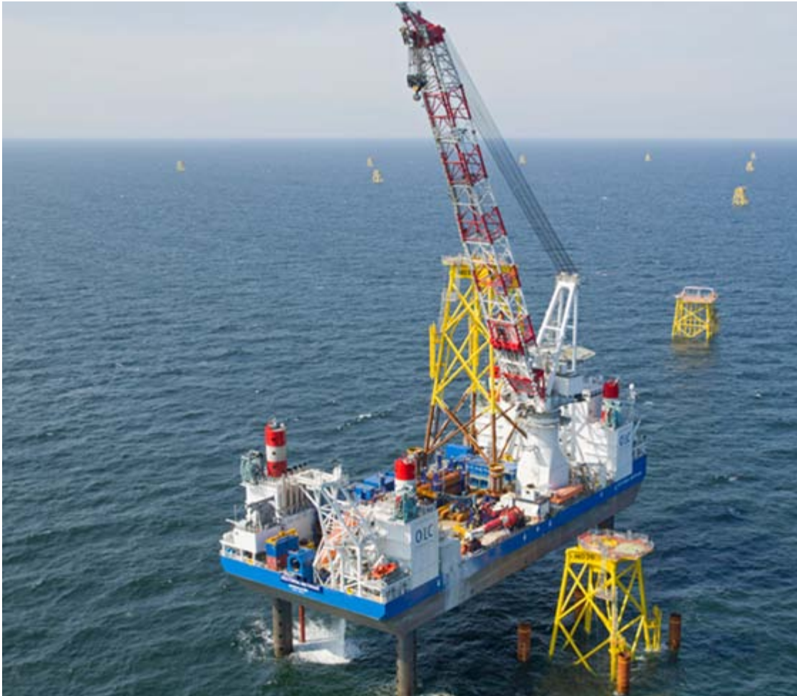
The VICTORIA MATHIAS during installation of a jacket in Nordsee Ost Offshore Windmill Farm north of Helgoland.
