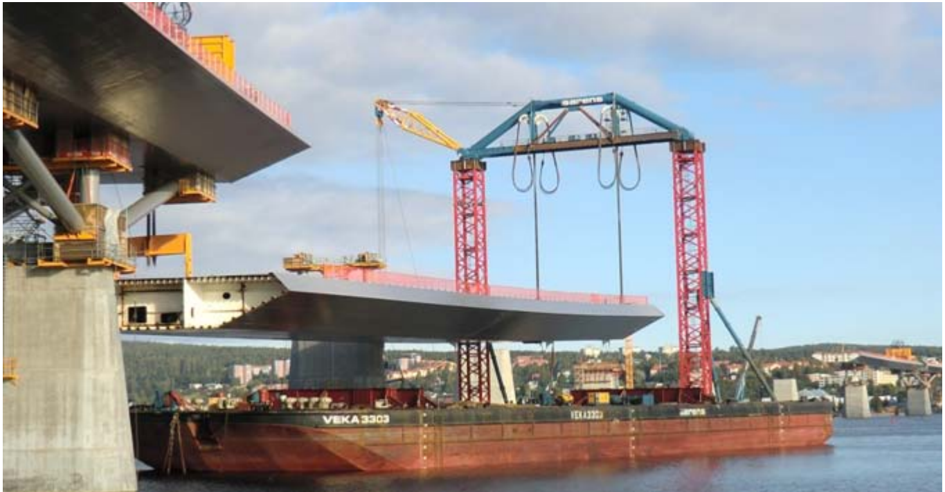
Last Saturday the 4th bridge section (length 132 mtr, weight 2010 T) over Sundsvall's bay in Sweden was installed by SARENS . Behind the transport barge VEKA 3303 , the WIM/TOM TWINBARGE was situated with a lifting gantry. – Photo : Max Bögl ©
