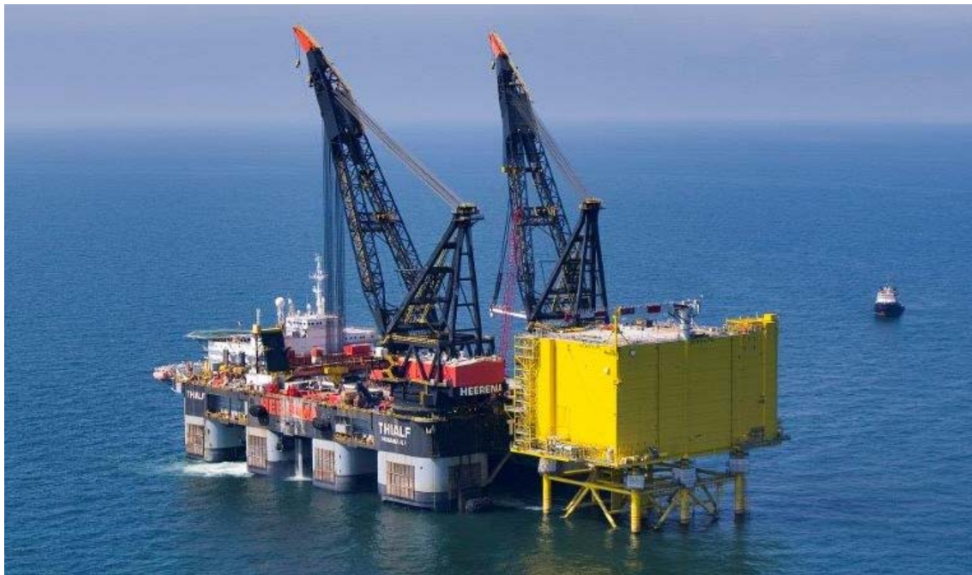
The Heerema fabricated DolWin Alpha was installed by the THIALF at it's position 75 kilometres out into the German North Sea Photo : Tom van Stenis ©
