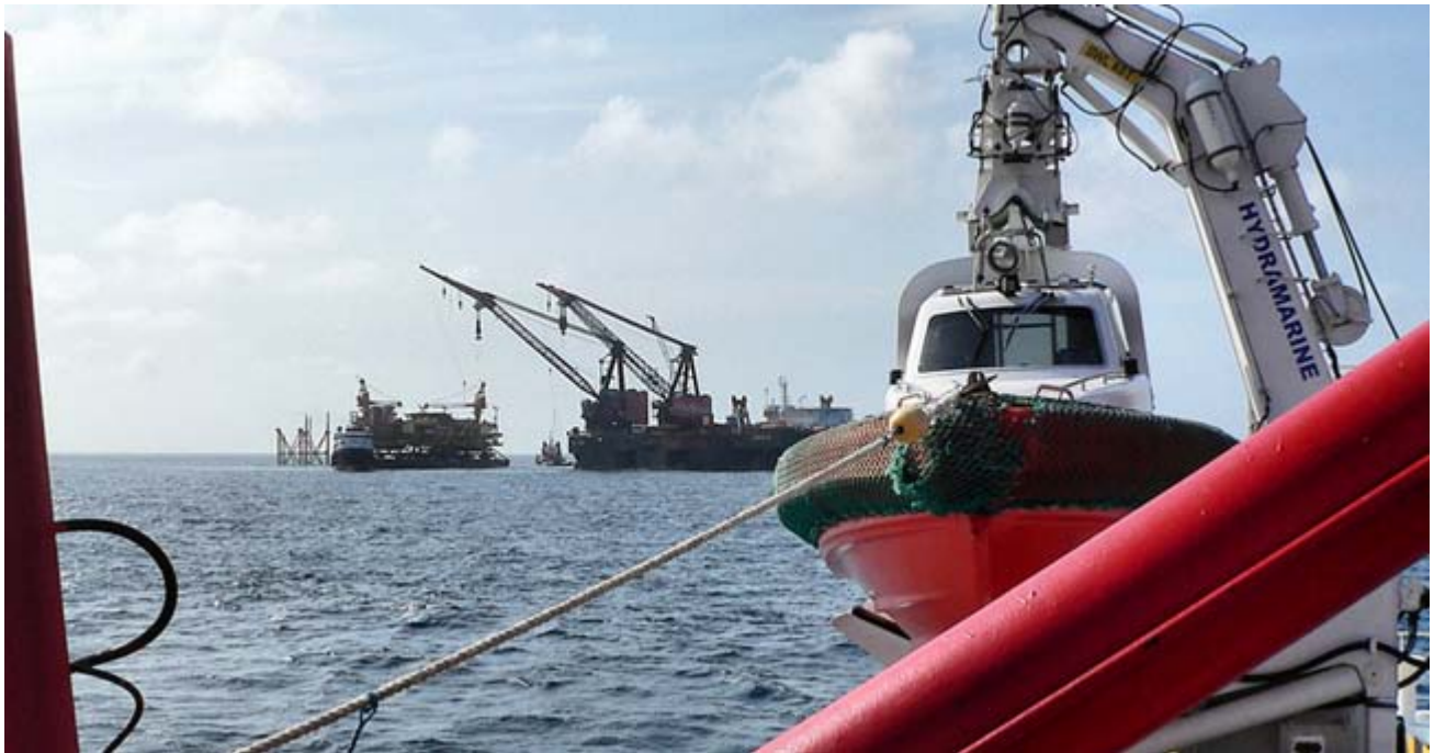
The HERMOD with BYLGIA and RETRIEVER working together to place accommodation module on new West-Franklin platform as seen from the OCEAN TROLL – Photo : Ch.Eng Iemke Kooijman ©
