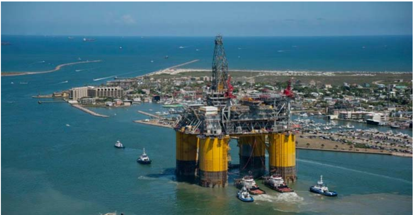
Above seen the tow-out of Shell's new built TLP platform Olympus . The tow-out took place on July 13th with very tight clearances on the sides and bottom with 6 Signet tugs and 2 Crowley Ocean Class new built tugs. A total of 20.000 hp was pushing the hull via the la Quinta channel with 9 mtr clearance each side out to the seabuoy on a beautiful day. Hundreds of spectators were along the towroute to watch it leaving the channel.
