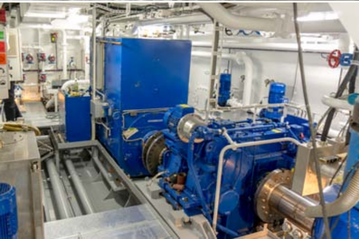
as well the 2 engine rooms , with above seen one of the shaft generators
