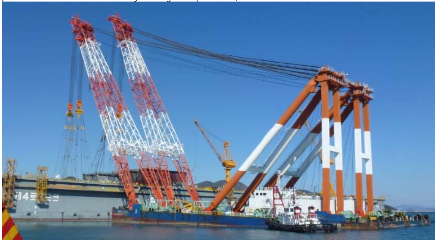
Large floating crane at DSME in Okpo lowering a large section in the newbuilding dock – Photo : Piet Sinke ©
