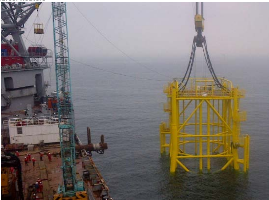
The OLEG STRASHNOV installed the Meerwind jacket – Photo : Joop Waeijen (c)
