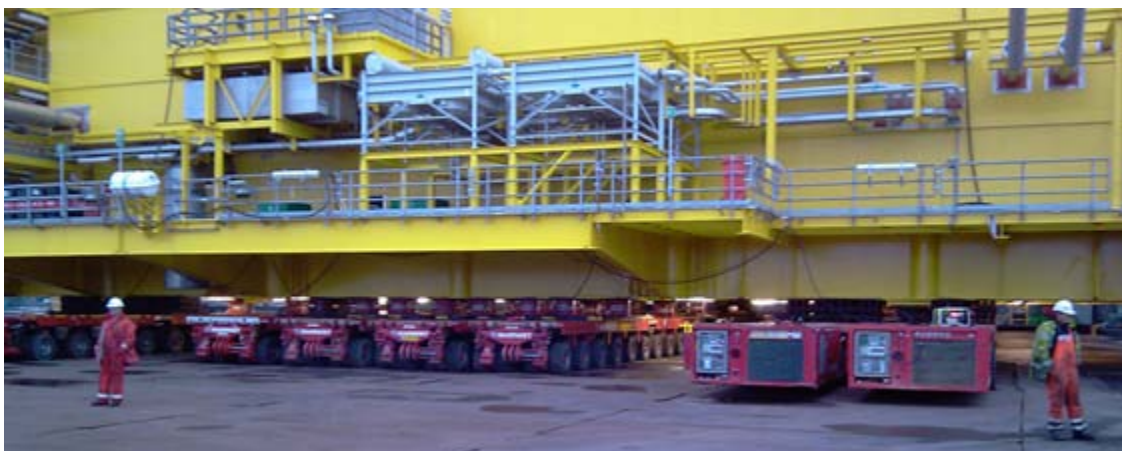
At the Heerema Fabrication Group yard in Zwijndrecht the 9300 tons module Dolwyn Alpha , was loaded out at Saturday 18-05-2013 Photo 's : Julien Mos ©
