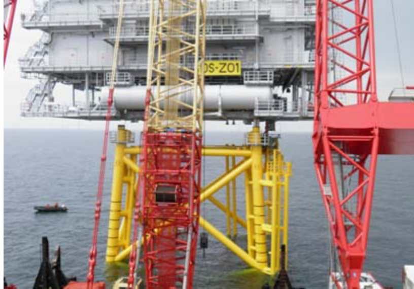
Installation of Topside Wods Substation on 16-05 Photo's Capt.Arno C ©
