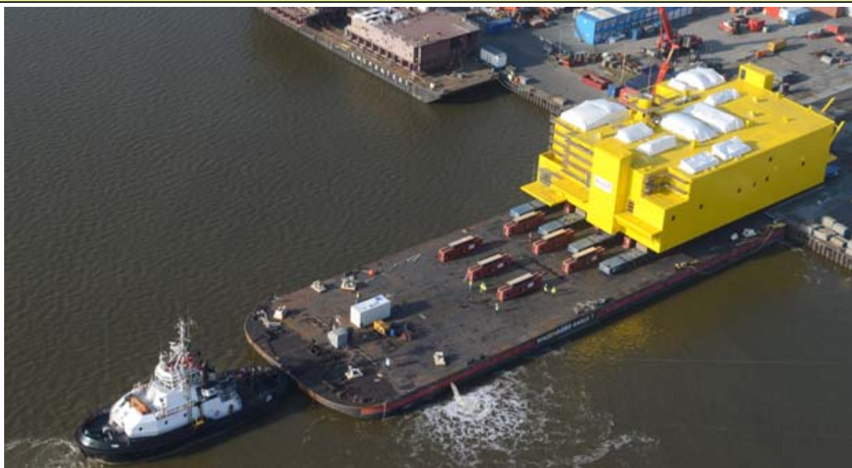
The load out of the transformator platform 288 MW onboard the Wagenborg 7 barge in Bremerhaven for the Meerwind project Photo : Joop Waeijen ©
