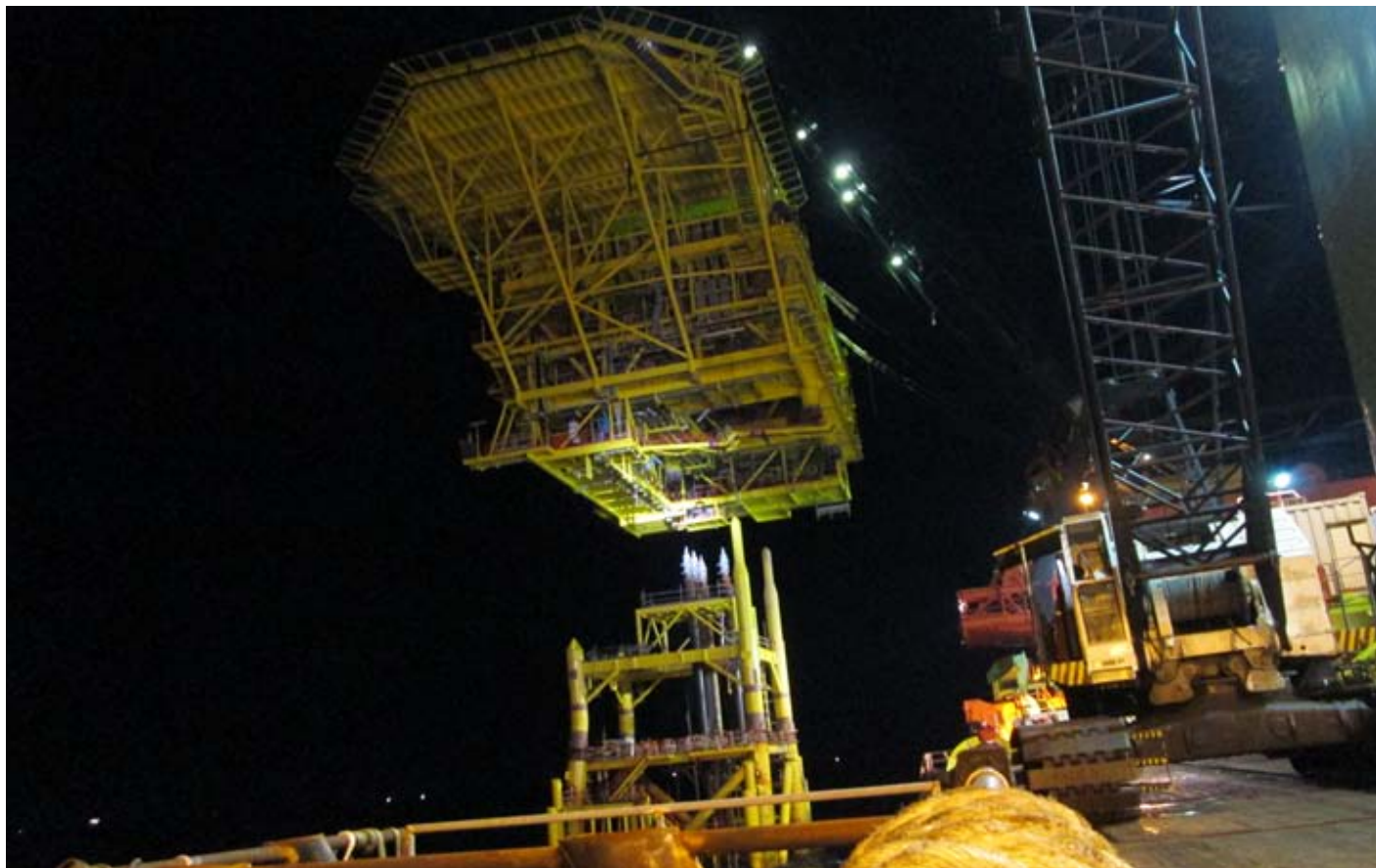
DLV CASTORO OTTO performing heavy lift of 1650 Tons topside Hai Su Trang WHSP offshore Vietnam.
