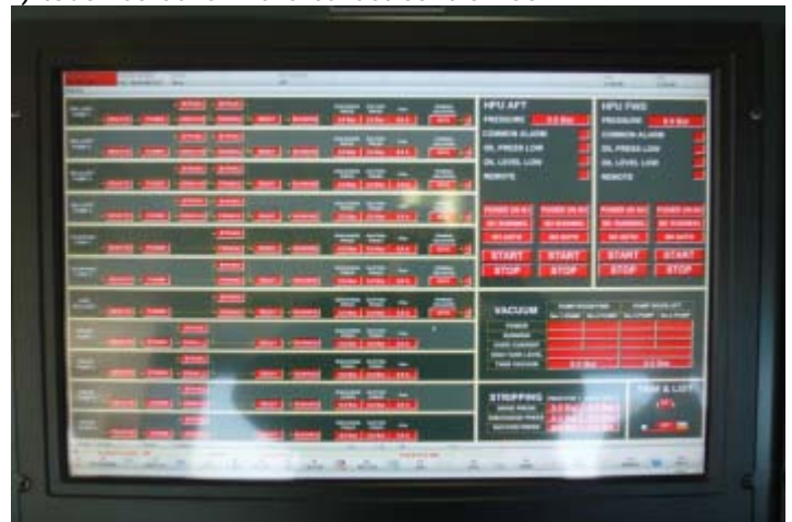
The ultra modern Ballast panel with all large (27 ") touch screens in the ballast control room
