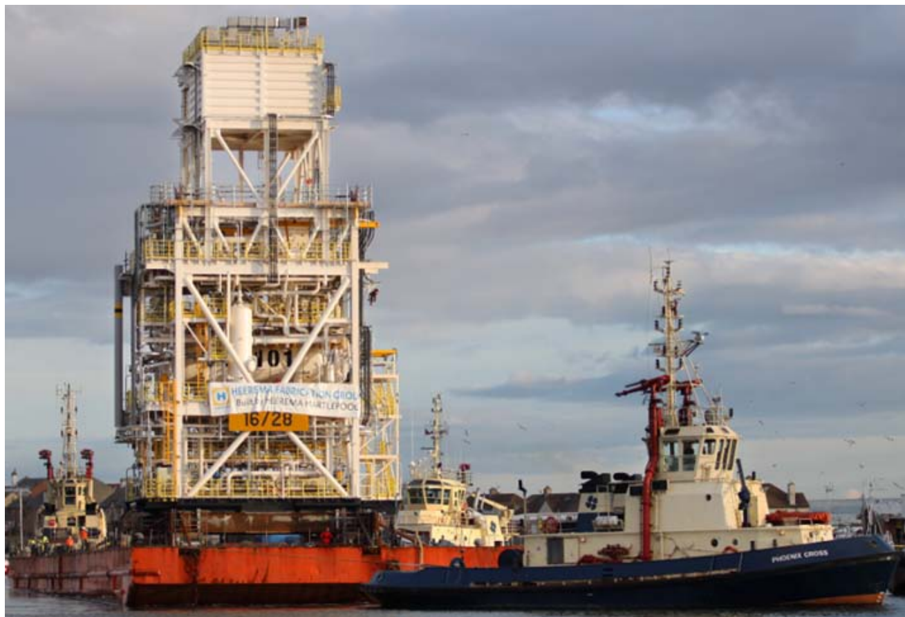
'Barge UR 108' departing Hartlepool with new build module onboard from Heerema' Photo : Nathan Hobday (c)
