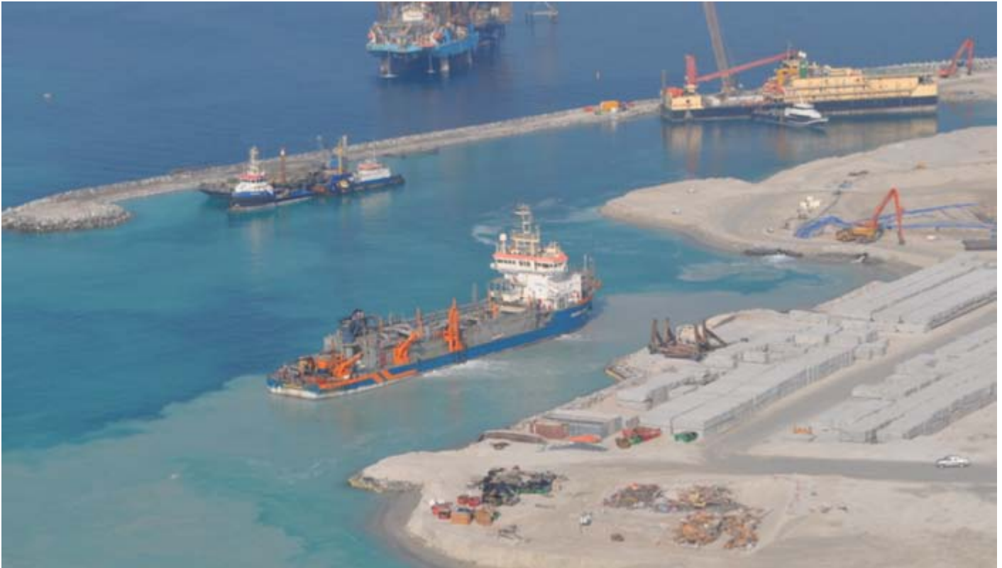
Birds eyes, Van Oords Volvox Atalanta during clean-up dredging in front of a quay-wall at one of the artificial island in Abu Dhabi waters- Photo : Maarten Mostert (c)
