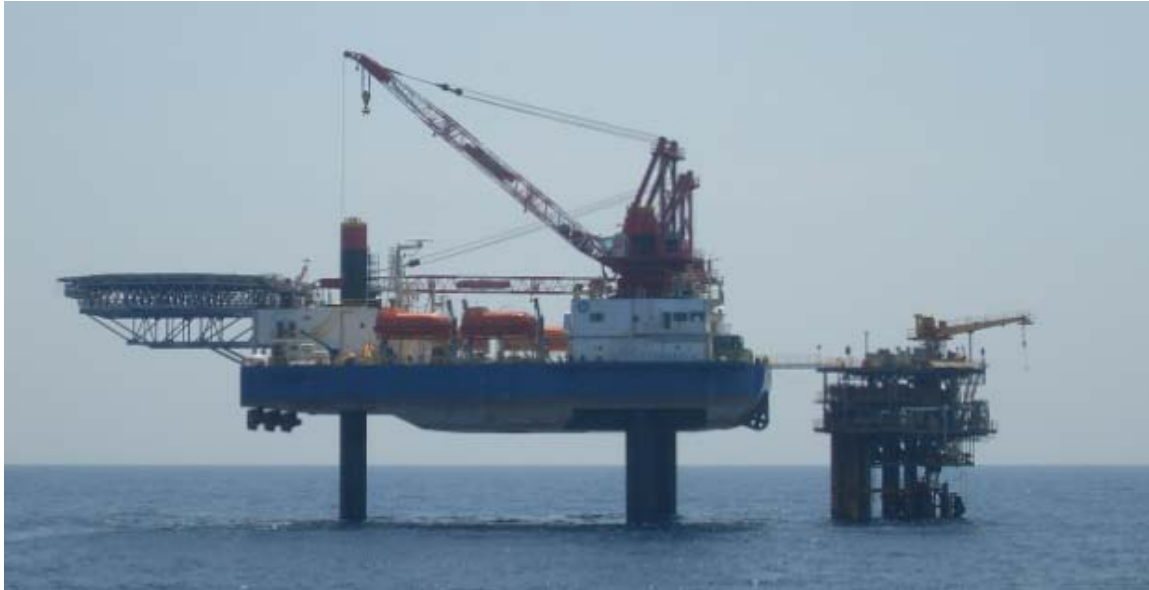
" Teras Conquest 6 " fully jacked up at the first platform location off Surabaya, with an air gap of just under 11 metres.
