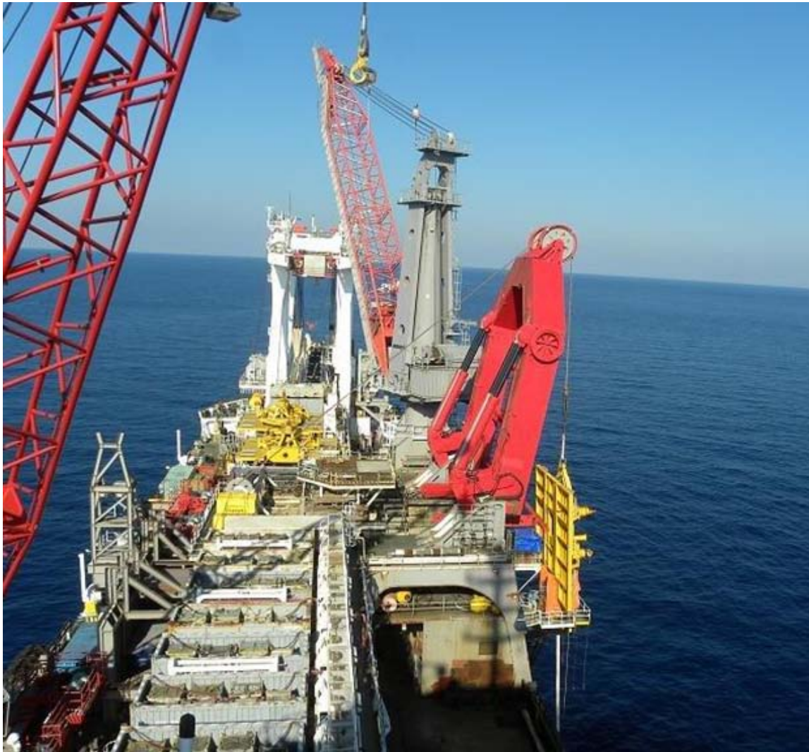
The PLV Audacia installing the FLET structures in J-lay mode on the 10 inch pipe in to the Mediterranean Sea for the Noble Tamar project offshore Israel. - Photo : Pieter Kos
