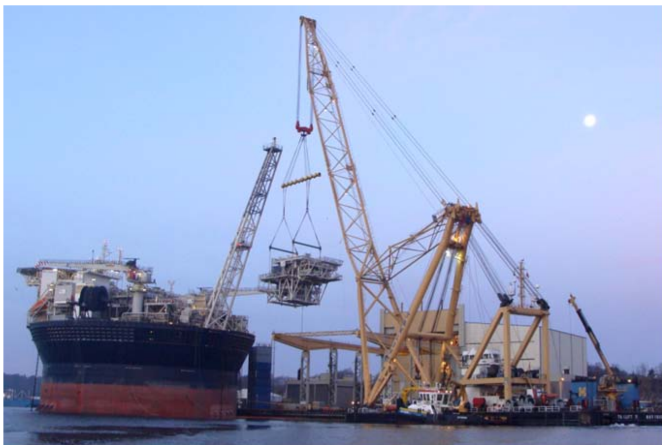
Last Sunday, Smit's sheerleg TAKLIFT 7 lifted a 430 ts module onto FPSO ' SEVAN VOYAGEUR ' at Eydehavn, Norway. This was one of several lift to be carried out onto the FPSO - Photo : Crew TAKLIFT 7 ©
