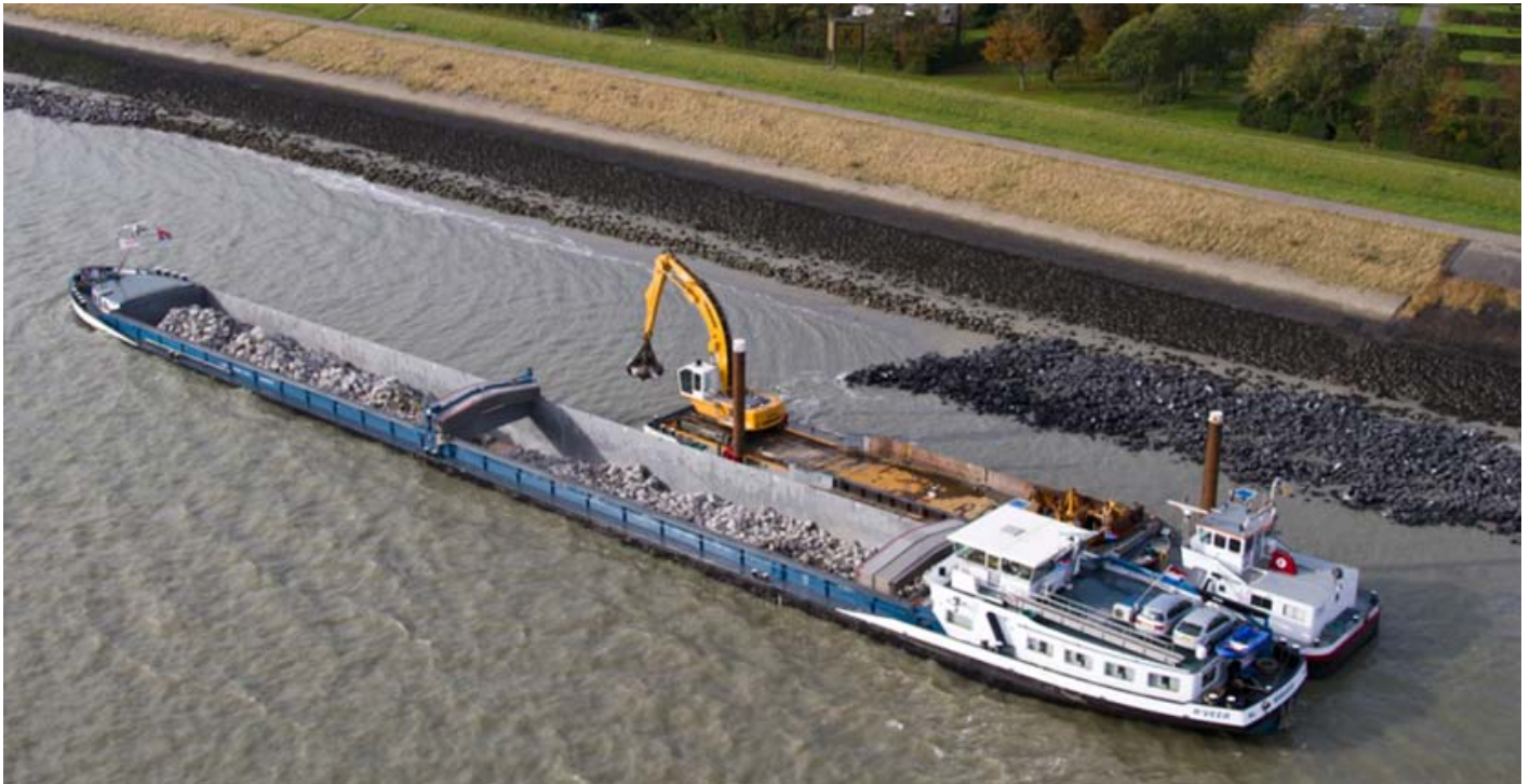
The Magri seen working for van Oord near Hoedekenskere, delivering rocks for the reinforcement of the coast line.
