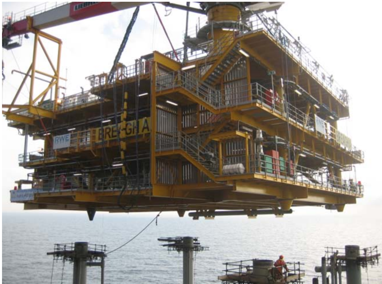
Above seen the Breagh A topsides during the installation at the jacket in the Northsea, the topside is built at Heerema Fabrication Group and installed by Heerema Marine Contractors last week Sunday ( October 16th)
