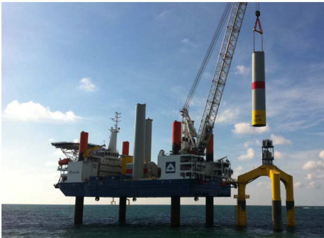
THOR seen building up tower S2-8 of BARD 01 Offshore windmill .
