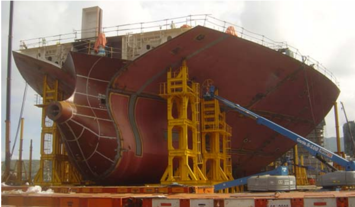
Stern section of a vessel under construction at the Samkang M&T shipyard in South Korea
