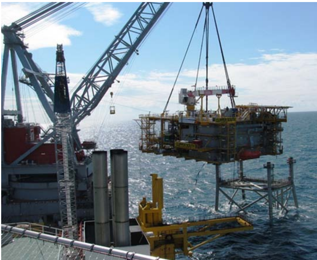
The OLEG STRASHNOV seen lifting the first Offshore Clipper South deck in the North Sea Photo : Adri & Smithy ©
