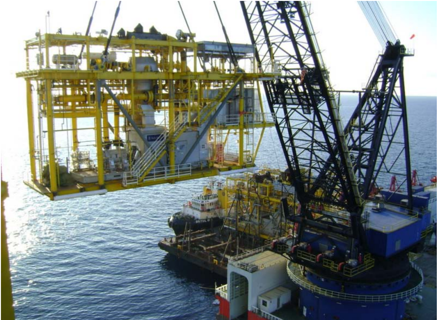
Above seen the DLB NorCe Endeavour installing compressor modules at PTT's Erwan field in the gulf of Thailand Photo : Cornelis Jagt - Solstad Offshore Asia Pacific Ltd (c)
