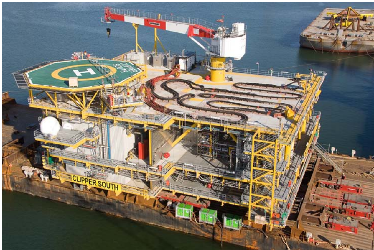
Last Friday at the Heerema Fabrication yard in Vlissingen the nearly 2400 ton CLIPPER SOUTH topside was loaded at the AMT VENTURER . The 80-0 tons jacket for the same platform departed 1 week earlier at the same pontoon under tow of the tug TEMPEST , The CLIPPER SOUTH jacket/topside is constructed for RWE Dea and will be installed at a location 70 km NE of Bacton (Norfolk), UK.
