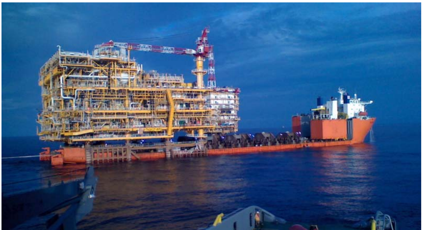
DOCKWISE BLACK MARLIN seen on the 13th of August, during the undocking phase after a successful completion of the float-over operation of the 19,500mt Bongkot 4A topside onto the PPS jacket.
