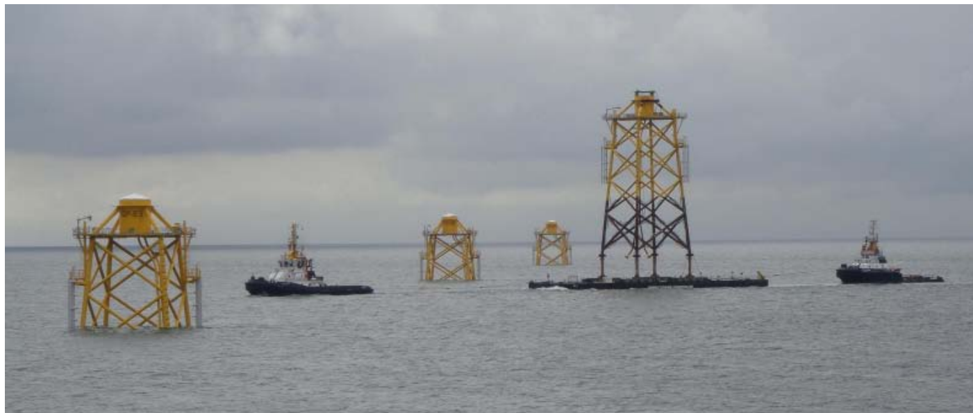
Approach of the " Union Grizzly " and " Union Sapphire " with a new jacket for the Thornton Bank, to be installed by HLV " Rambiz ". Photo : Capt Henk Doornhein – Master Rambiz ©
