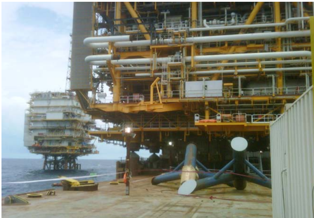
Above seen the Black Marlin while lowering the Bongkot PPS Topside onto the jacket during the Bongkot Float-over in the Gulf of Thailand. Photo : Erik van Empel (c)
