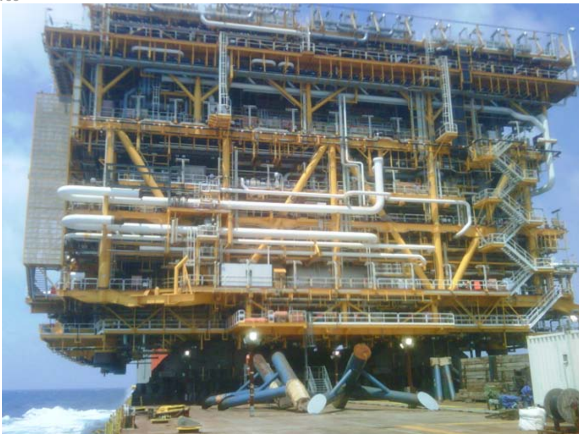
Above seen the Bongkot PPS Topside on deck of Dockwise BLACK MARLIN while in transit from Ulsan, Korea, to the Bongkot Field in the Gulf of Thailand in preparation of the Bongkot Floatover.
