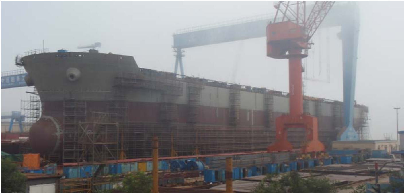
Above seen at the Cosco Dalian Shipyard a newbuilding with hull number 354 (Noble Shipping) and below a newbuilding for Vroon (Breskens – The Netherlands) the post Panamax bulk carrier SCOTIAN EXPRESS seen fitting out. The 51,209 GRT SCOTIAN EXPRESS is having a length of 229 mtr and beam of 38 mtr, and is powered by 1 MAN – B&W 6S60MC main engine of 12,240 kW for a top speed 13.7 knots - Photo's : Clemens Smits ©
