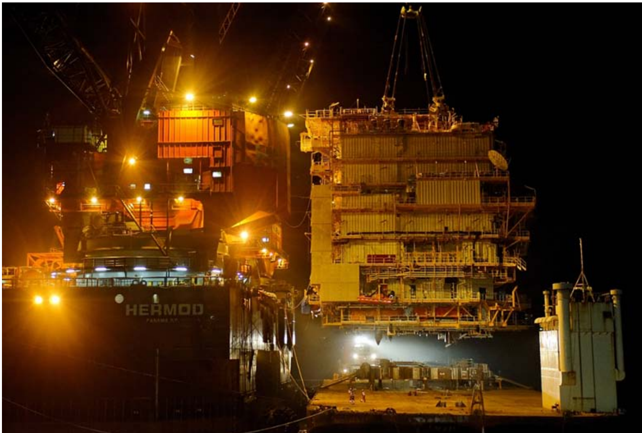
Above seen Heerema's HERMOD seen lifting the 4000 tons (in weight) Bongkot QPS module - Photo : Capt. Jan Berghuis ©
