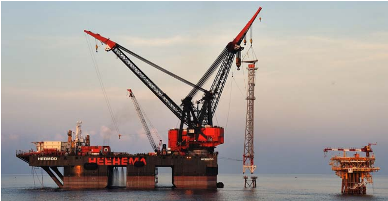
The HERMOD seen installing the flare tower on Bongkot Field - Photo : Capt. Jan Berghuis – Master Husky ©
