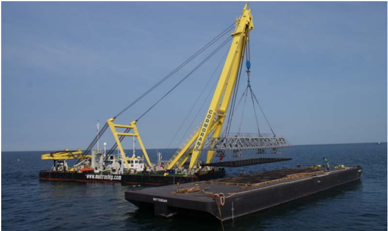
Multraships CORMORANT seen installing mats at the Thornton Bank project Photo - Wout Kamerman - Multraship (c)
