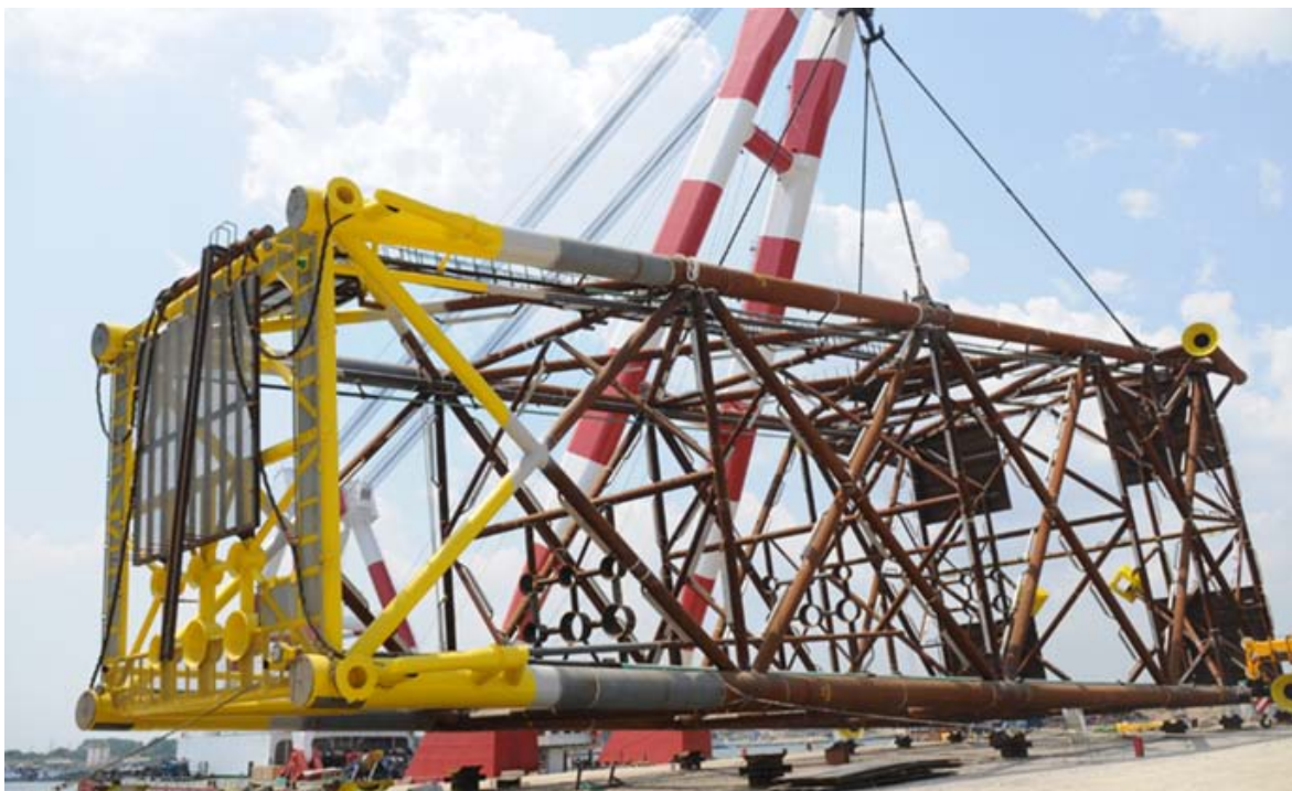
Seen at the GSP SHIPYARD CONSTANTA ROMANIA the load out of a 101 mtr long and 1300 tons jacket ready for transportation to Akcakoca /turcia - Photo : Neagu Nicolae Daniel ©
