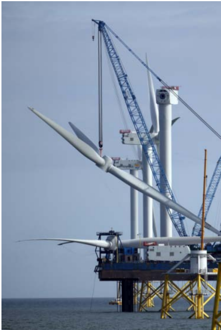
Above seen the SeaJack lifting blades at the Ormonde windfarm Barrows UK.
