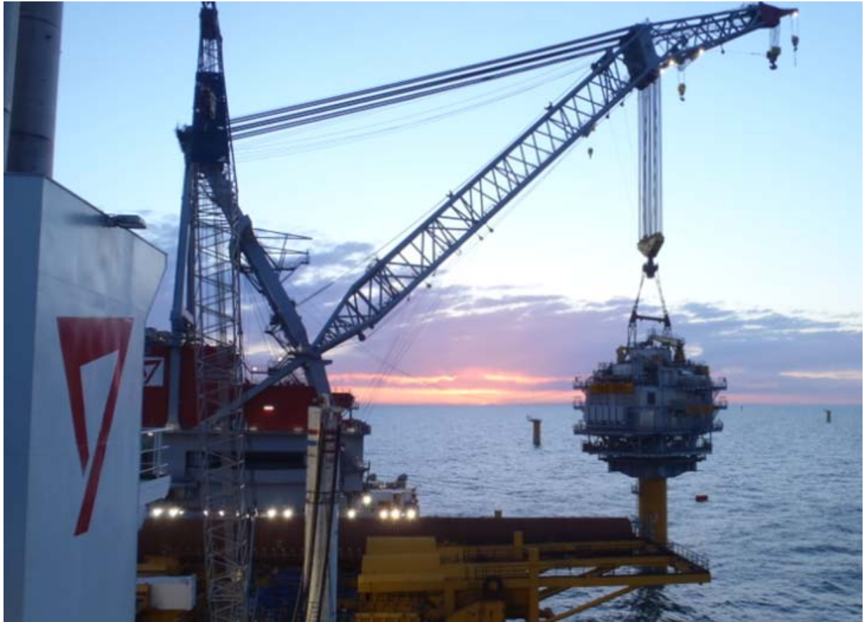
The OLEG STRASHNOV seen installing the Substation OS1 in the Sheringham Shoal Wind Farm Photo : Peter Hollander (c)
