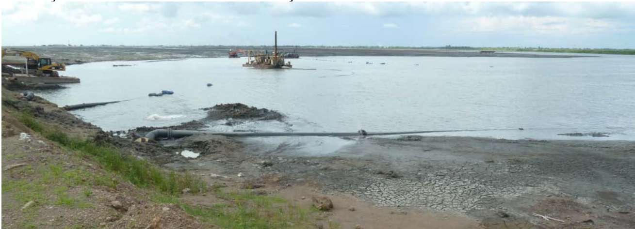
The mud is pumped by small dredgers into the Porong River at present – Photo's : Piet Sinke (c)
