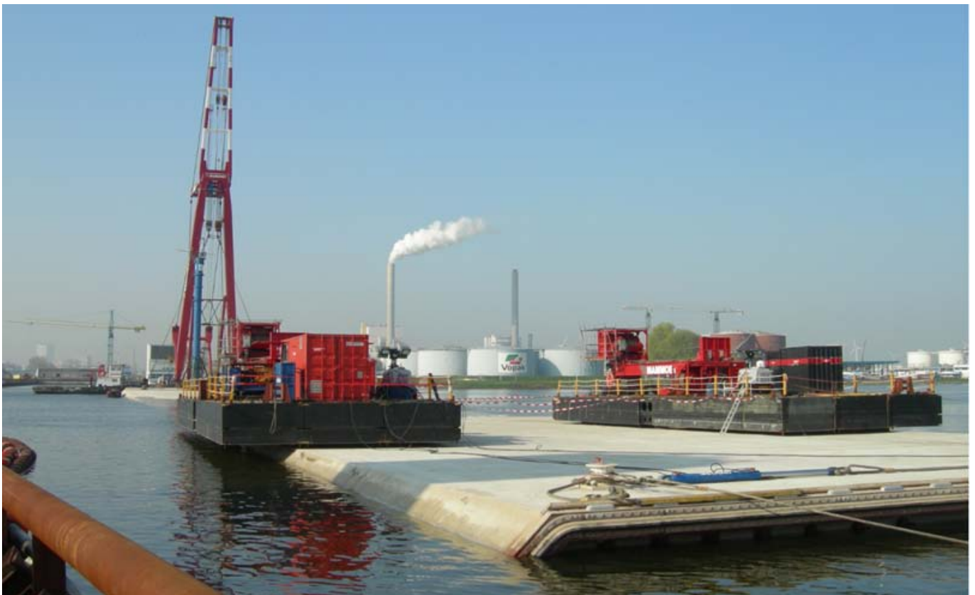
Last Monday (18-04-2011) tunnel element TE-3 of the new 2 nd Coentunnel was submerged into final position, Photo's : Jos Leentvaar - MAMMOET Maritime B.V. ©
