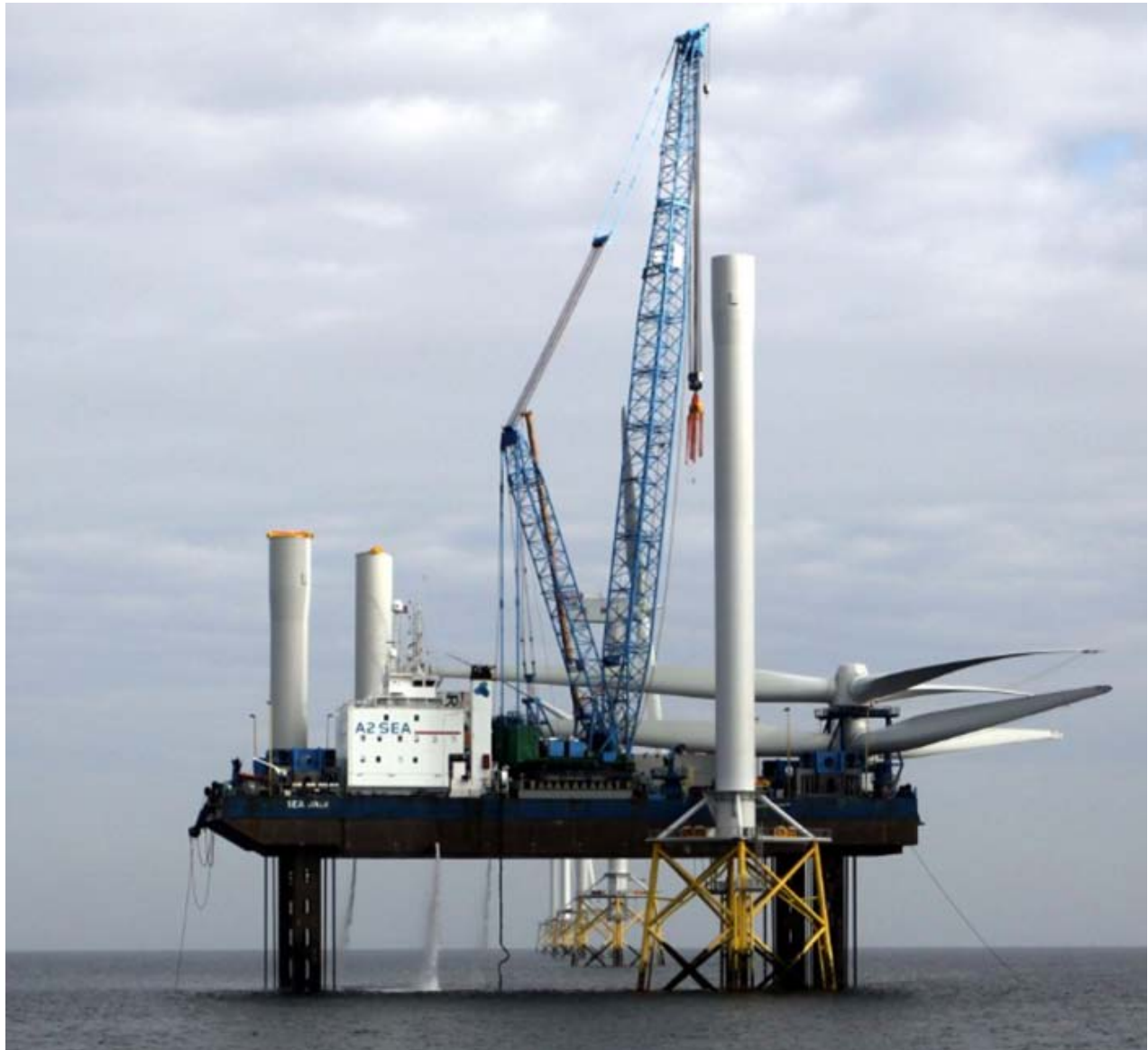
The SEA JACK seen installing Wind Turbines at the Ormonde field bij Barrows UK
