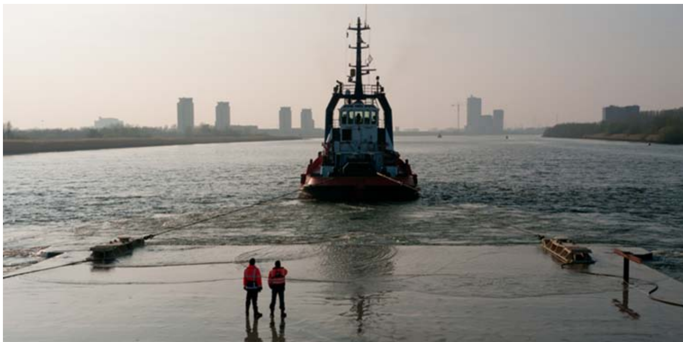
Tunnel element no 1, the last element for the new to built 2 nd Coentunnel was safely transported from Barendrecht to Amsterdam – Photo : Marijn van Hoorn ©
